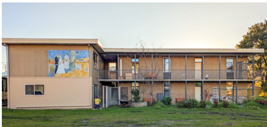
The refurbishment of the Zoe Flats has given new life to a building with a long connection to Morwell and St Luke's Uniting Church.
